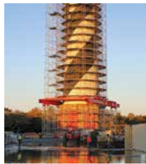
Cape Hatteras Lighthouse Buxton, NC
