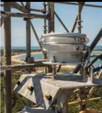
The exterior light installed on the scaffolding around the lighthouse.
