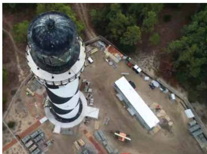
Drone view of Cape Lookout Lighthouse Stabilization Project. Cement foundation laid around the apron of the Lighthouse. Scaffolding is going to be added soon.
